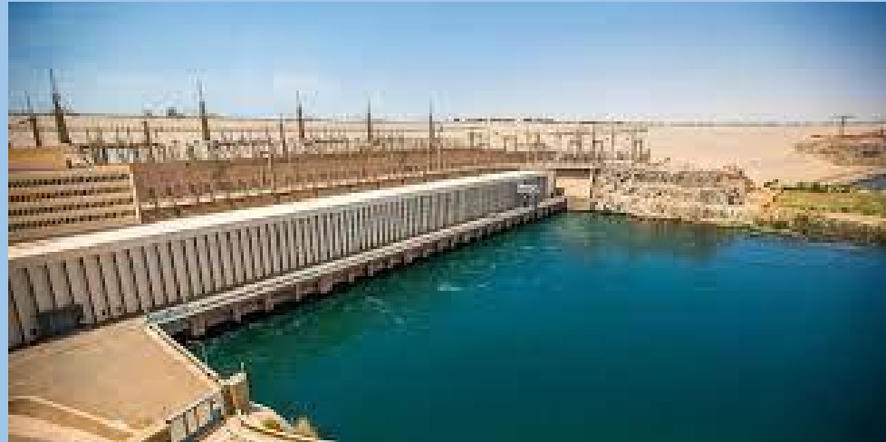
The Aswan High Dam
